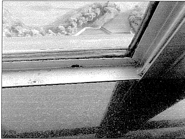
21 – IGU in 1470 building
