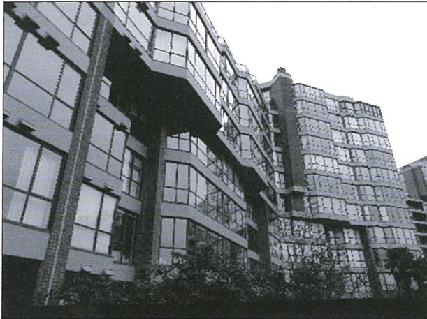
16 – Windows overlooking east courtyard
