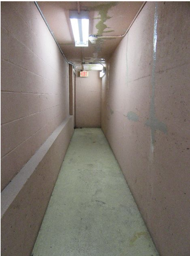
37 – Parkade exit corridor
