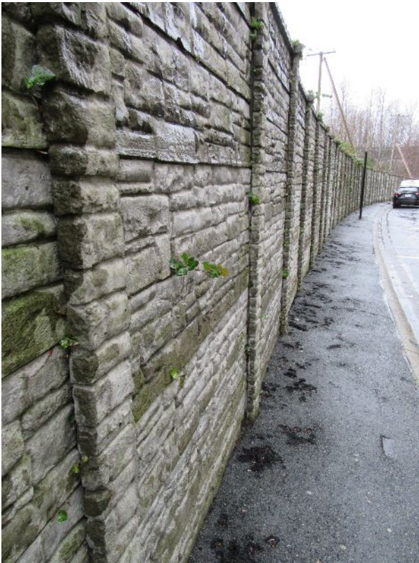
62 – Precast concrete fence
