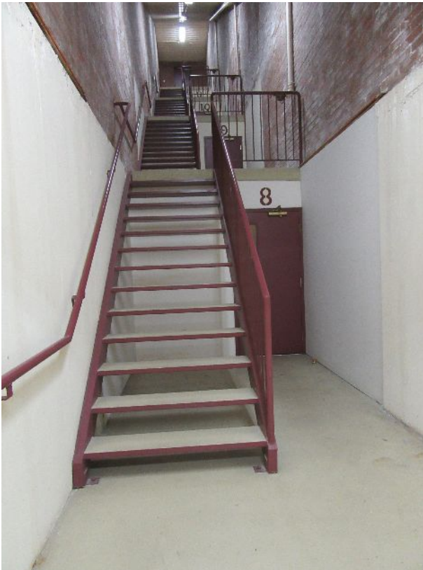
38 – 1450 stairwell (Stair No. 2)
