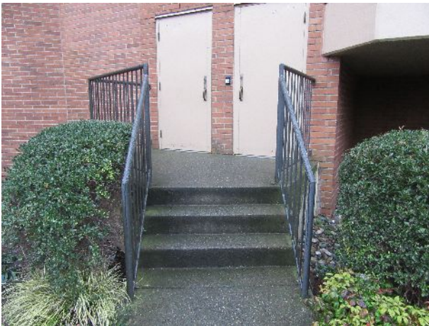
71 – Guardrails at elevated stair landing
