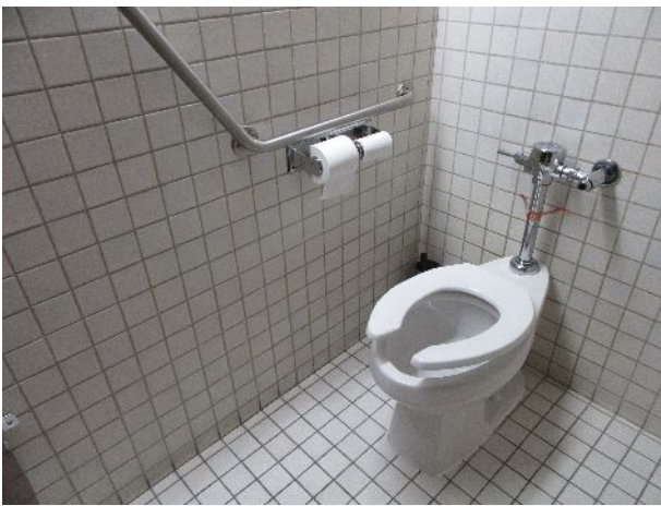
114 – Plumbing fixtures in men's change room
