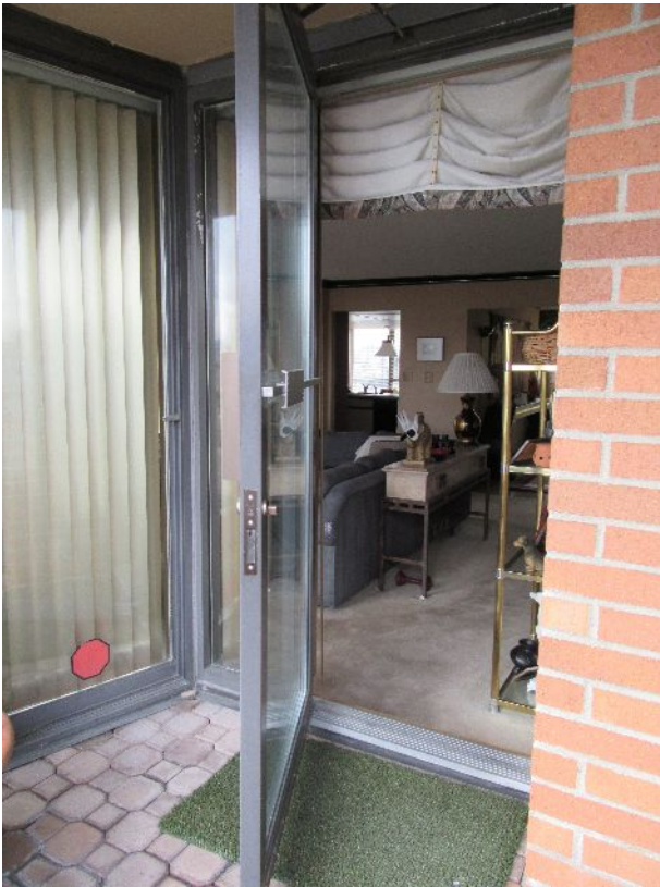
23 – Aluminum-framed swing door at 1450 roof deck
