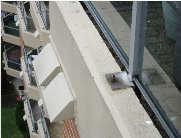
28 – Painted concrete upstand and vent hoods
