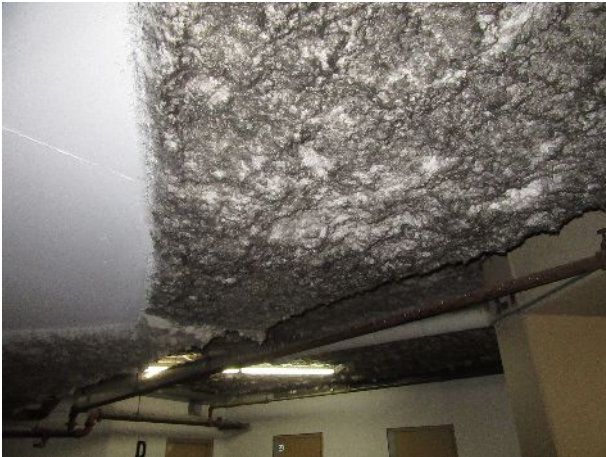
138 – Spray-applied insulation in parkade
