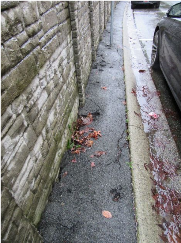
58 – Asphalt walkway west of Pennyfarthing Drive
