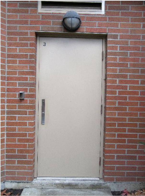
25 – Hollow metal exit door
