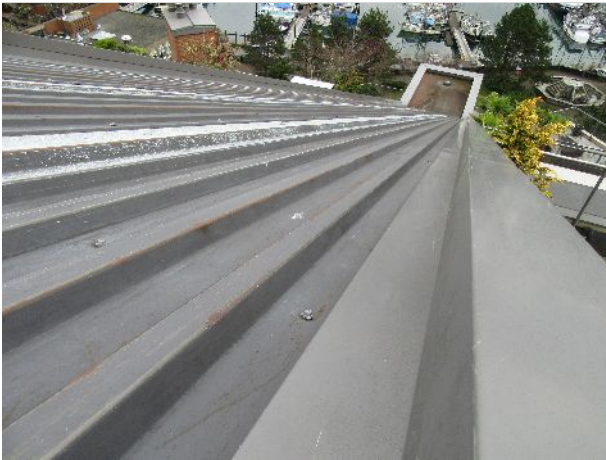
5 – Metal roofing over 1450 stairwell
