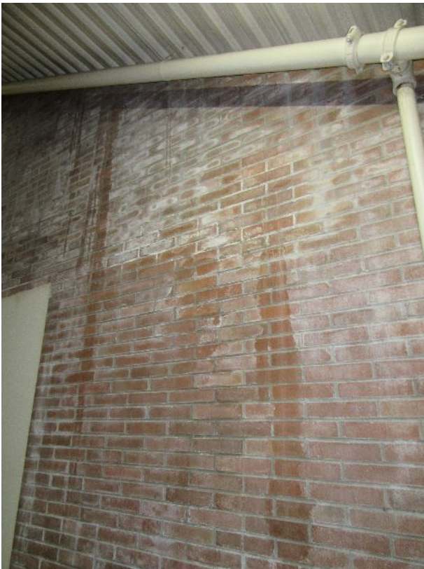
14 – Structural clay brick wall in 1450 stairwell
