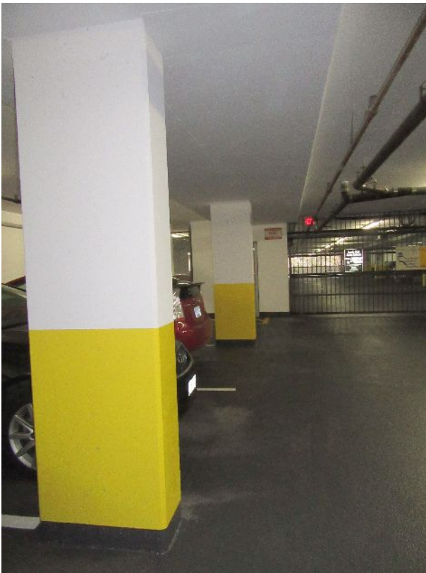
145 – Slab band supported by concrete columns
