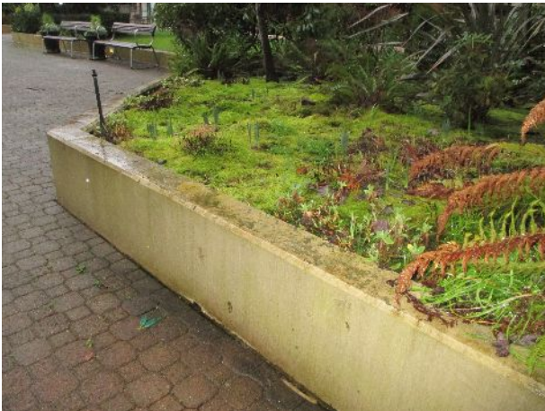
66 – Concrete retaining wall in east courtyard
