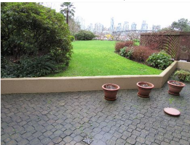
67 – Concrete retaining wall around patio
