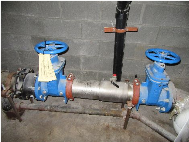
109 – Double check valve assembly
