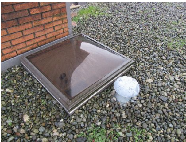
3 – Acrylic dome skylight on 1470 roof
