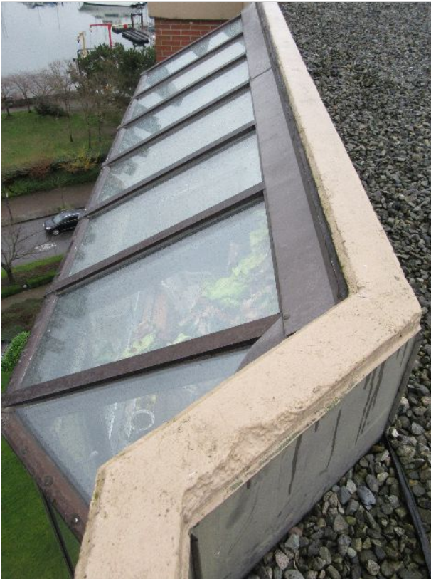
19 – Solarium skylights at 1490 building
