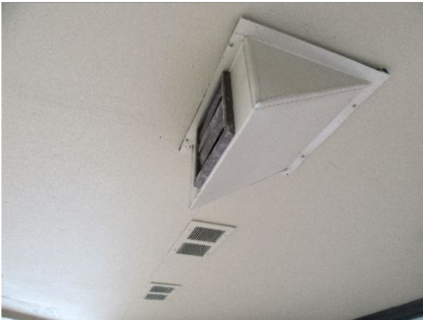
29 – Painted balcony soffit
