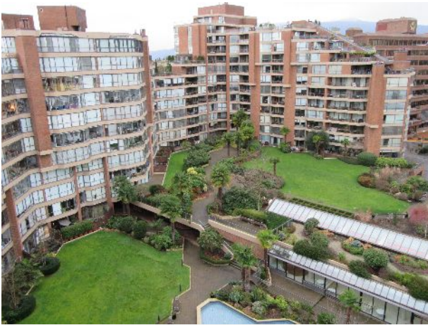
56 – Exterior grounds over waterproofing membrane
