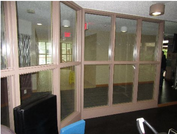
44 – Glazed interior partition at exercise room
