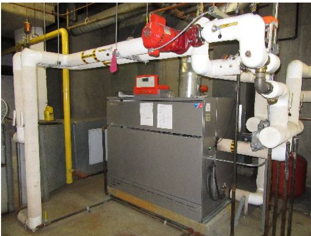
118 – Viessmann pool and hot tub water heating boiler
