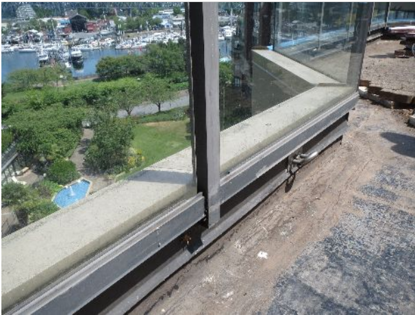
7 – Exposed roof deck membrane (2015)
