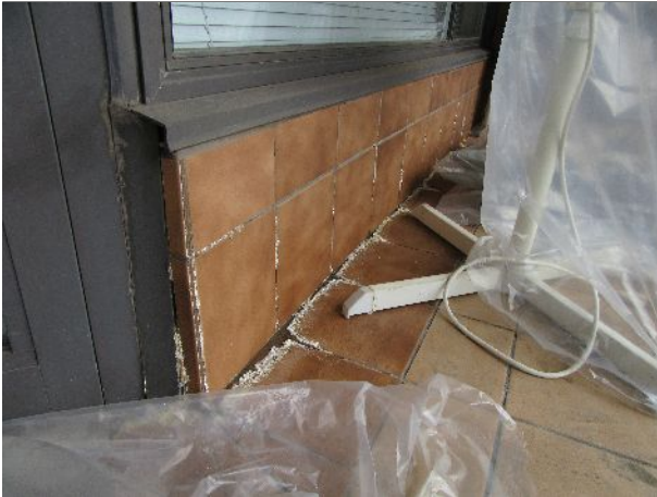
10 – Tiled wall below balcony window
