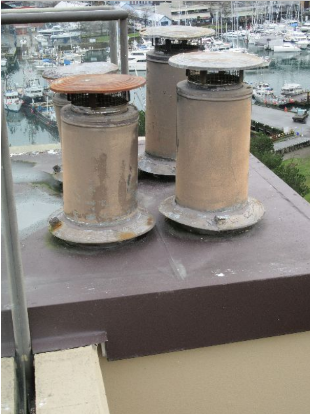
106 – Gas flues at top of chimney
