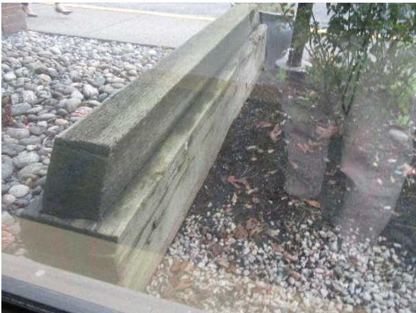
69 – Wood retaining wall on west elevation
