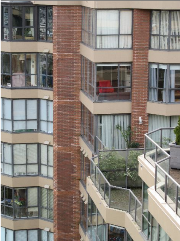
13 – Past brick veneer repairs
