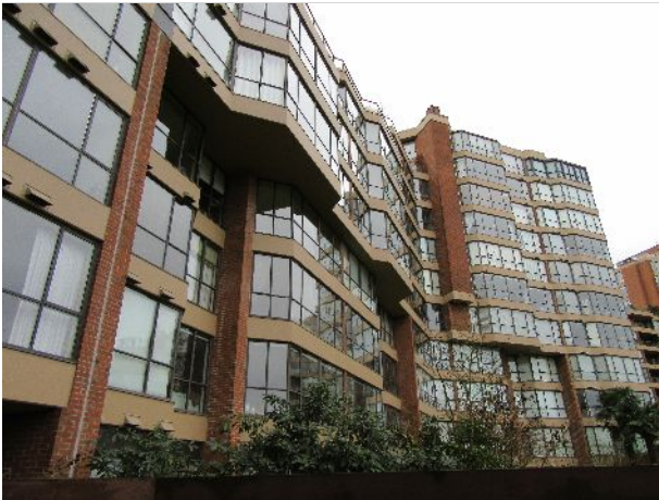
16 – Windows overlooking east courtyard
