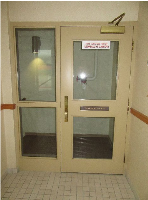
35 – Glazed metal stairwell door and sidelite
