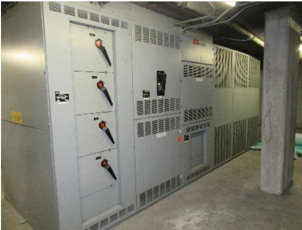
73 - 1470 unit substation
