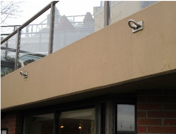
30 – Through-bolt anchors in concrete upstand
