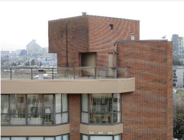
12 – Brick cladding at 1490 building
