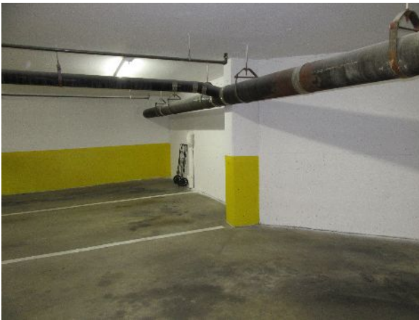
139 – Painted parkade walls and ceiling
