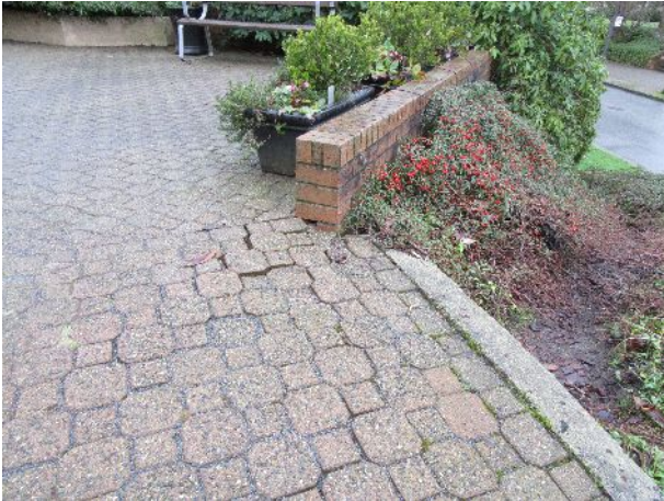
61 – Walkway close to Creekside Drive
