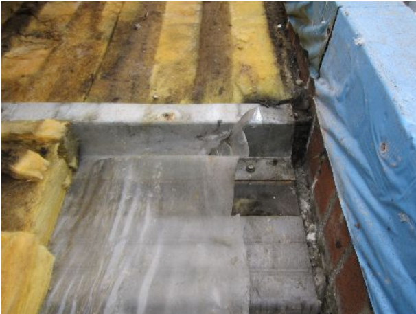
6 – Exposed metal roof assembly (2015)
