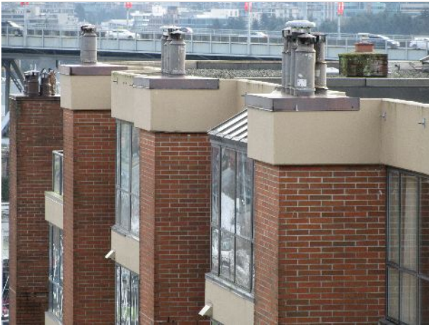
105 – Fireplace flues at top of chimneys
