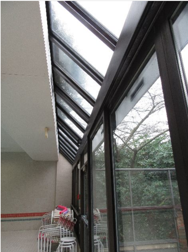
18 – Storefront glazing system of pool area
