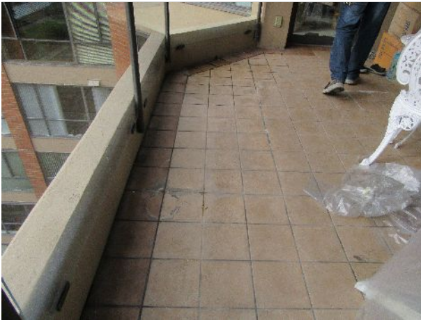
9 – Tiled balcony at 1450 building
