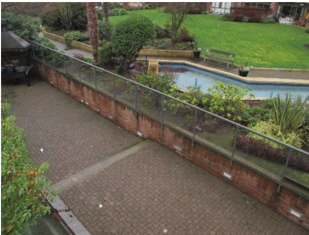
70 – Brick retaining wall at lower courtyard
