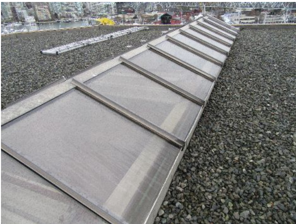
2 – Skylight over unit in 1490 building
