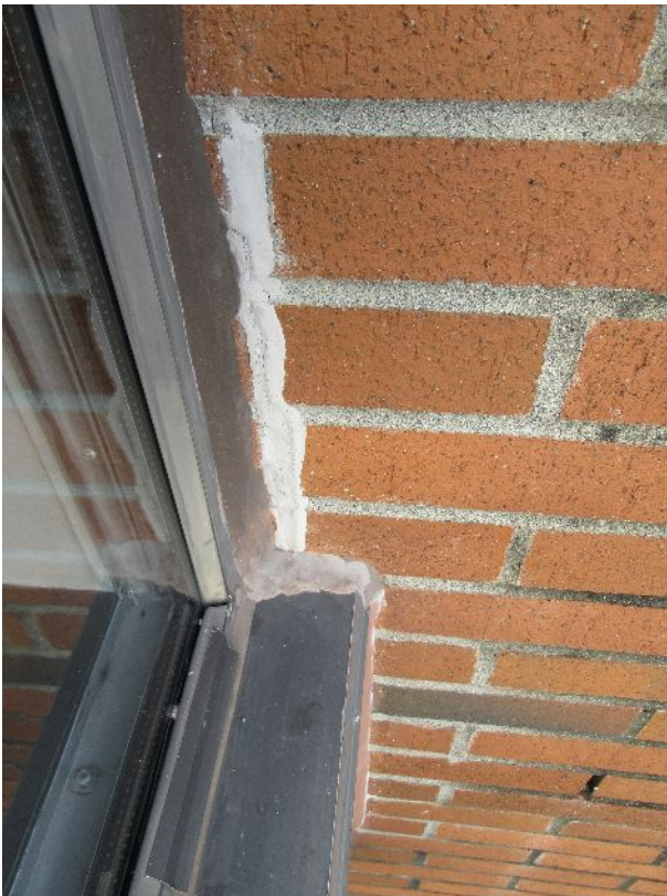
27 – Sealant at window-to-brick interface
