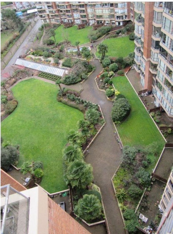
132 – Exterior grounds over parkades
