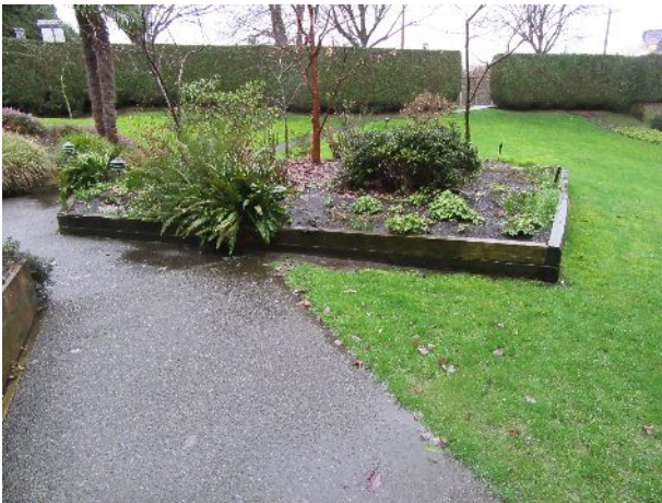
68 – Wood retaining walls at south courtyard
